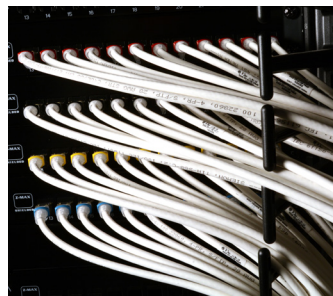
Smaller diameter cable significantly reduces bundle and pathway fill for space savings.
